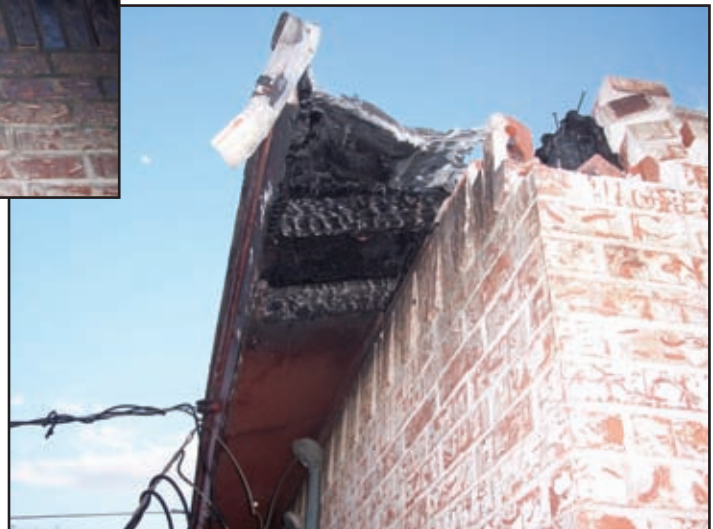
Grass embers entered through the gable vent on this house and ignited attic materials which resulted in the loss of the roof despite mitigation efforts by local volunteer fire departments.
