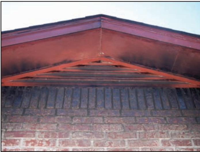
Grass embers entered through the gable vent on this house and ignited attic materials which resulted in the loss of the roof despite mitigation efforts by local volunteer fire departments.
