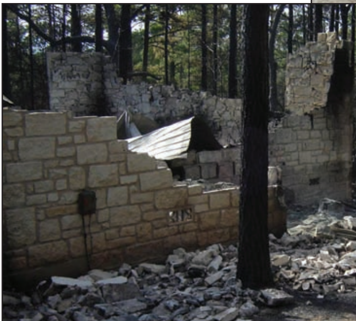
Despite the masonry construction, foundation vents allowed the entry of embers and flames into the home.
