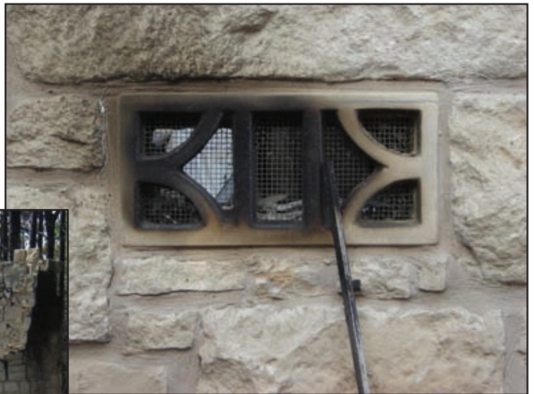
Despite the masonry construction, foundation vents allowed the entry of embers and flames into the home.
