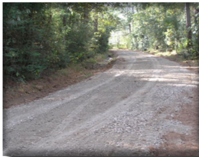
Rock is an excellent choice for roads that remain wet for extended periods of time or for roads with a high erosion potential.
