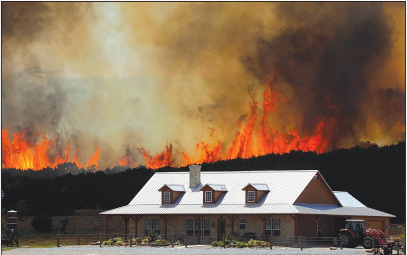
**This home was constructed with fire-resistant materials — masonry siding and noncombustible roofing — and used Firewise landscaping practices that greatly increased its survivability and created a safer working environment for firefighters.**
