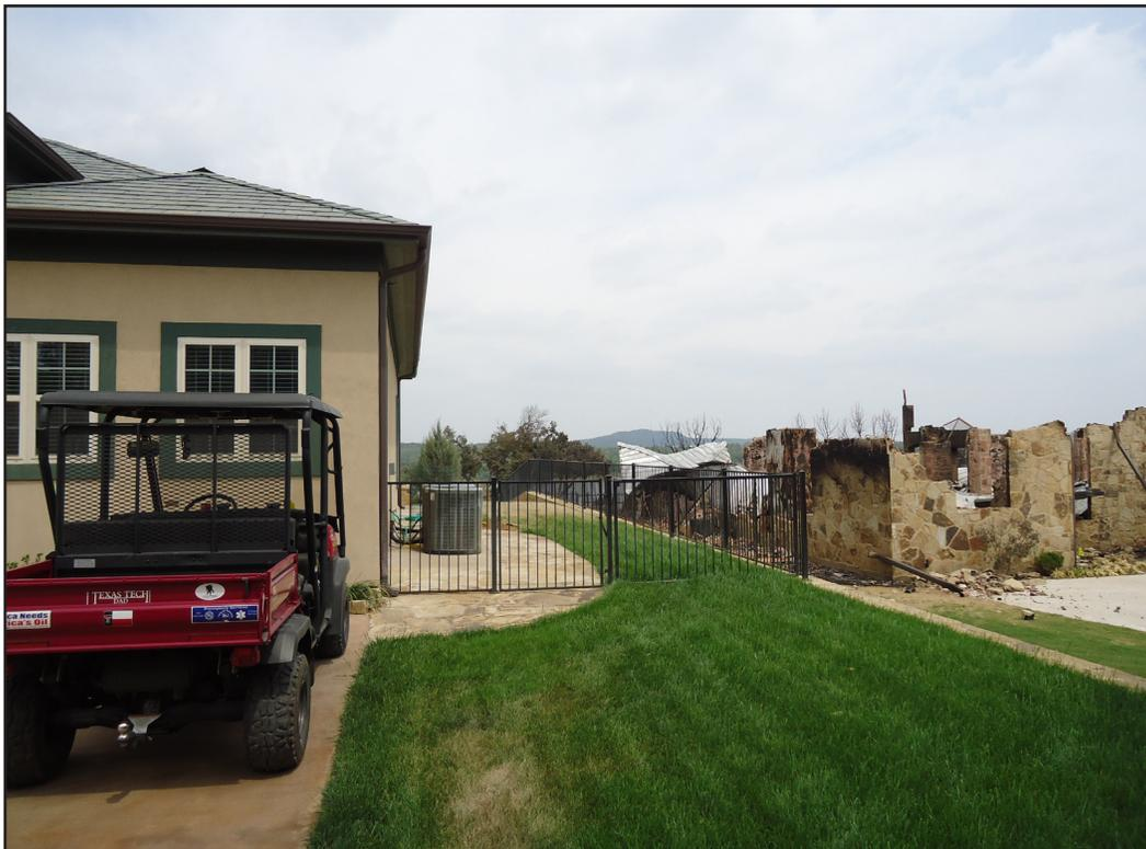
**The tiered landscape, elevated retaining wall, irrigated lawn, gravel fire break and non-combustible wrought-iron fence likely provided additional protection to this home.**
