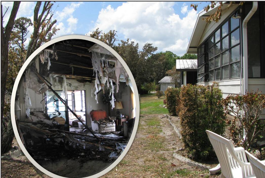
Embers from a nearby fire gained access to this home's interior, igniting it and causing significant damage.
