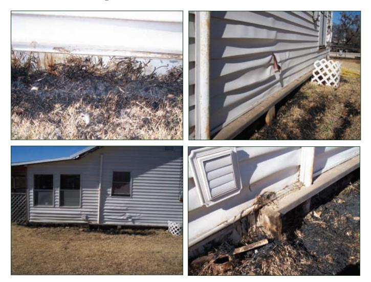
The homeowner stated that wind shifts from west to north brought the fire to the house. The fire department initially started suppression. Observations noted fire brands being carried by the wind to the side of the house and dropping them into the grass. Grass growing up under vinyl siding ignited, and consequently, the heat began to melt the siding and ignited the lattice on the back of the home.
