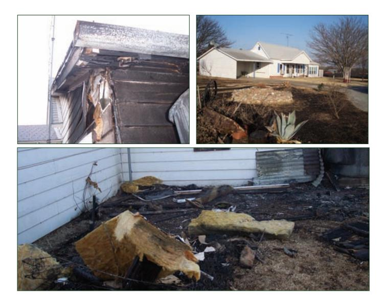
Despite numerous spot fires observed around the front of the home, ignitions actually occurred on the backside of the home. The large amounts of debris within close proximity to the home are credited with contributing to the ignition of the home.
