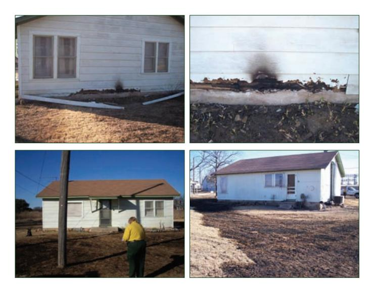
Dog runs on the front and back side of the home created a fuel break, keeping the fire from making contact on three sides of the home. Fire traveled to the side of the home where the dog's movement was restricted, allowing the fire to come in direct contact with the wood siding home. Radiant heat was significant enough to compromise single-pane windows and melted vinyl blinds.
