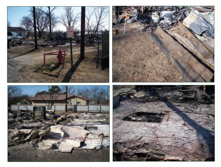
Landscape railroad ties carried the fire to the home and ignited the wooden beam foundation. Also, blown embers under the open foundation resulted in multiple points of exposure. Despite close proximity to hydrants, loss of the home occurred due to lack of manpower.
