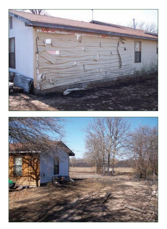
The lack of a break in fuels allowed the fire to burn directly to the side of the structure and melt the vinyl siding. The homeowners were forced to evacuate, but family members returned after the initial fire front passed to continue suppression efforts, saving the home.
