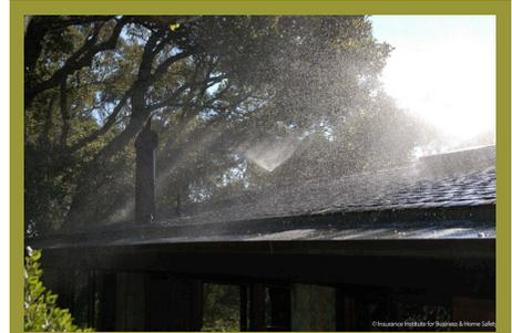
**Photo 1.** Roof mounted sprinkler.
