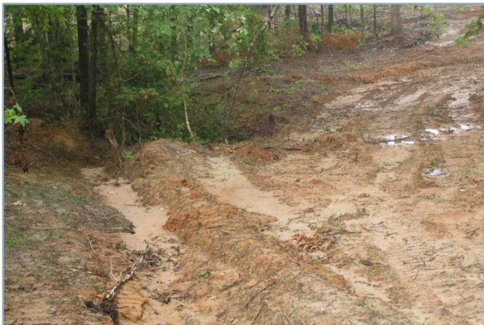
*Waterbar improperly draining into stream.*
